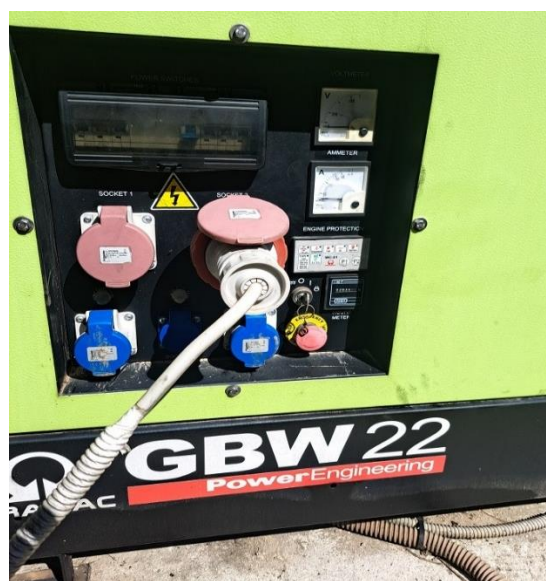
12. Agregat Pramac GBW 22 Y.M.C.P. diesel
