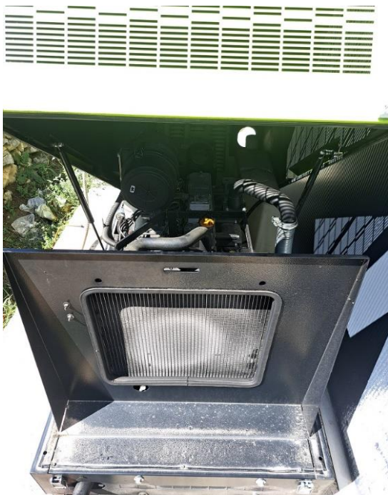
13. Agregat Pramac, radiator
